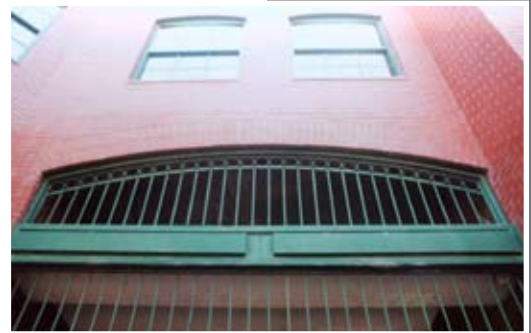
A strong railing design works well with the simple lines of the architectural façade.
