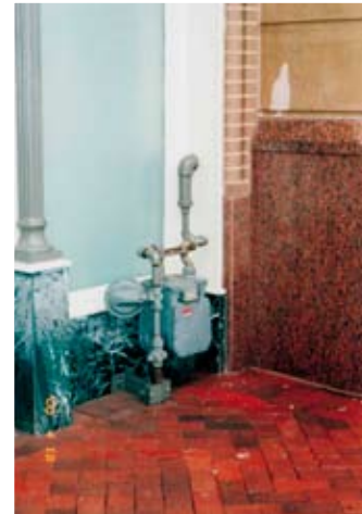
Utilities should not be exposed at the sidewalk because they run the risk of damage.
