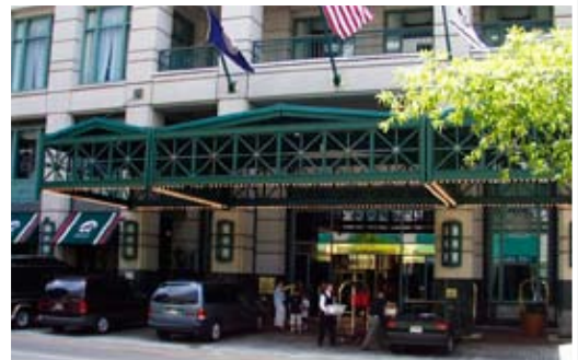
A building canopy can serve as a visual amenity as well as shelter for building occupants and pedestrians.
