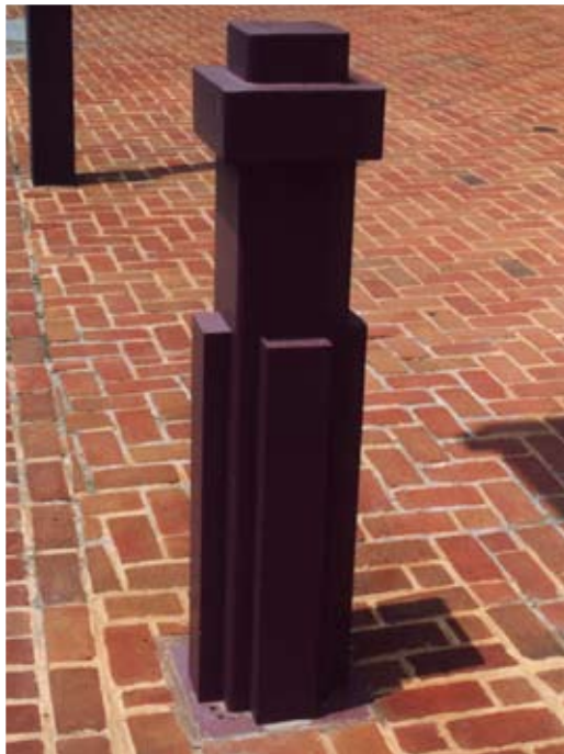
Metal bollards should be treated to resist the deteriorating effects of the elements.
